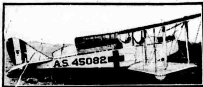
Every squadron in the army air service soon will be equipped with airplane ambulances like this, built at Dayton, O. The stretcher is in the fuselage and a special compartment is provided for a physician.
