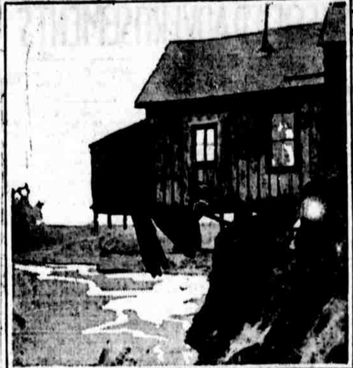
An example of the freakish activity of the waters that flooded Pueblo, Col. The kitchen of this house is hanging over the embankment without any support, except the long beams that reach out from the part of the house left on land.
