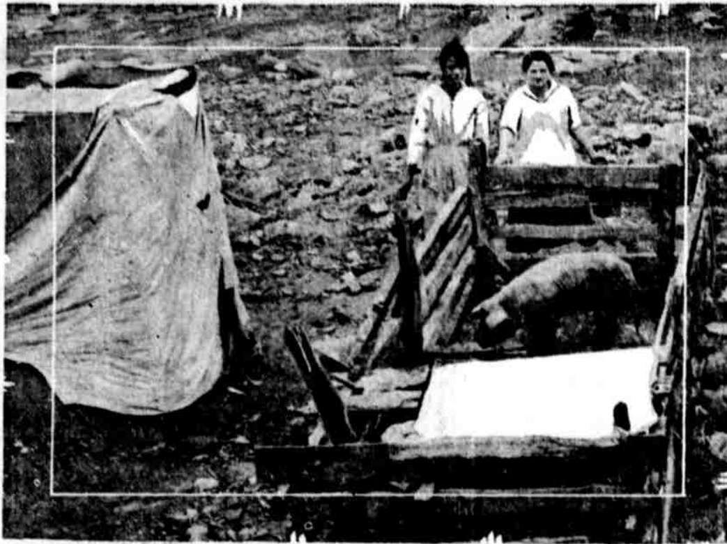
WILLIAMSON, W. Va., Dec. 28.—How the striking West Virginia miners are facing the severe cold weather is shown by this picture of a typical striker's home and his winter meat supply. This particular miner is more fortunate than most of the strikers—few have pigs. On the left is his shack, made partly of boards, partly of tenting, little bigger than the pig pen. The strikers' right to unionize is fully supported by the Miners' National union, which is sending supplies.
