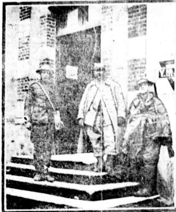
Thirty shrapnel holes in this 'Y' hut near Chateau Thierry testify to the heroism of the Y. M. C. A. workers in France. The building does not look like the picture for this photograph was taken before the German forces approached Chateau Thierry.
