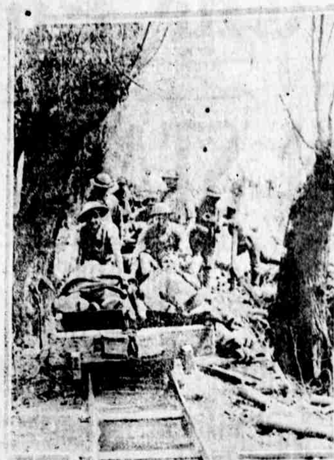
The transportation of the wounded from the front is one of the most serious problems of the military authorities, and the most logical plan yet devised is via the light railway. It is constructed at very low cost and can be shifted at will as the tide of battle changes. Many of these railways are now being used.
