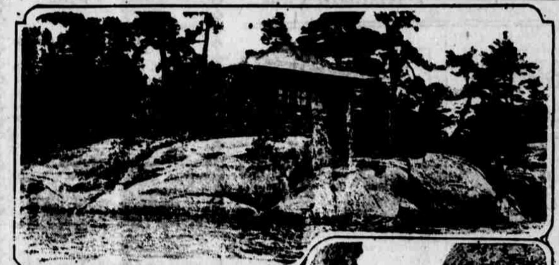
Play House at Point au Baril, Ont.
