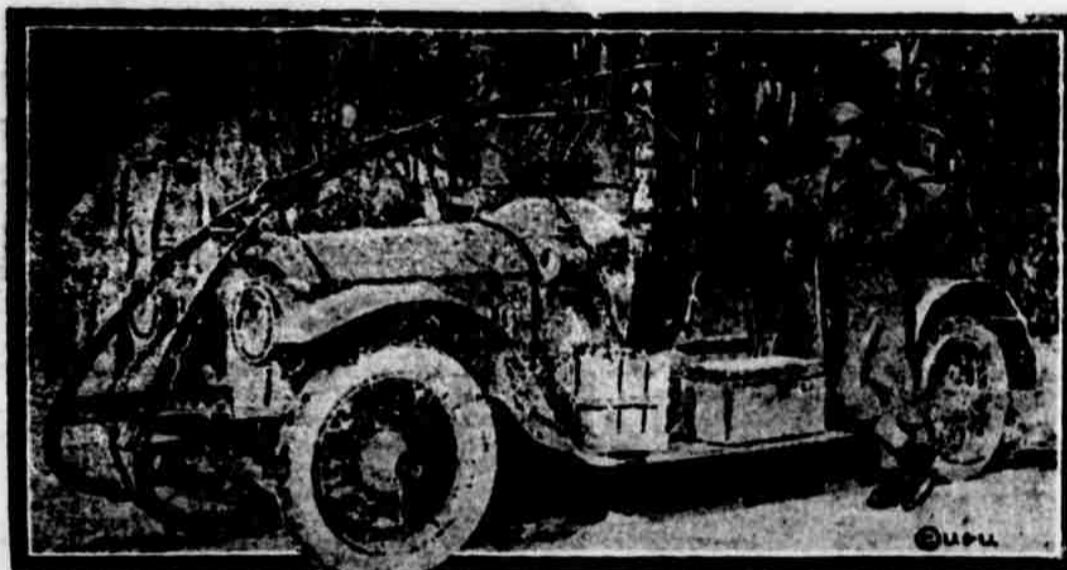
This is only another illustration of how carefully the Germans prepare for the war. The auto with a steel frame running over it is used to cut barbed wire entanglements in "No Man's Land" where they interfere with assaults over the trenches by their troops. The parts of the steel frame are so sharpened that the cut wire quickly and leave way for the soldiers to follow without injury.
