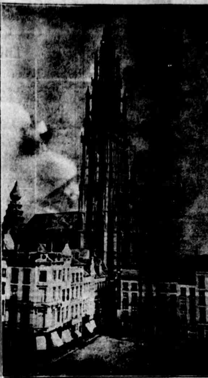
The Belgians who hurried from Notre Dame, which is one of the chief ornaments of the city. Though some bombs from Zeppelins were dropped near, none of them, so far as known, damaged the building.
