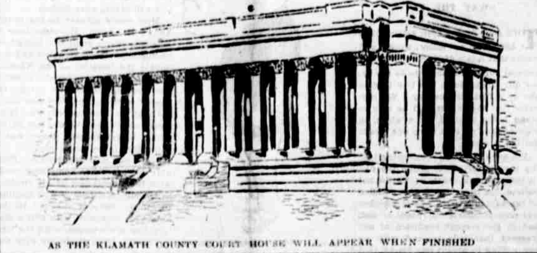
AS THE KLAMATH COUNTY COURT HOUSE WILL APPEAR WHEN FINISHED
