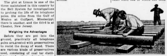
This borer will bring out a solid plug of wood which shows how far the creosote has penetrated the pole.
