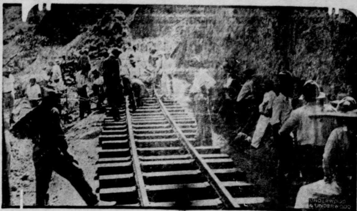
Fred Lavis, president of the new railroad, laying the rail in the road from the republic of Salvador, to the International Railways of Central America, bringing the country into direct communication with the Atlantic ocean. American engineers laid out the route and native laborers followed with steel, ties and rock. The 50-mile $12,000,000 link between San Salvador and Guatemala is through rain forest and jungles.
