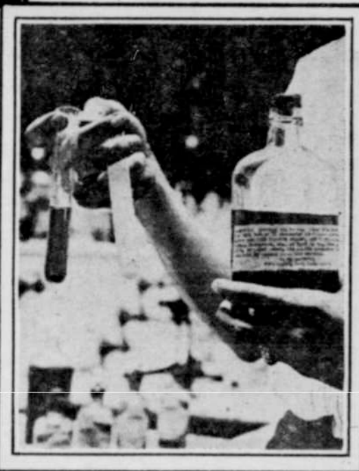
Photo shows an analysis of poison whiskey showing the sample of poison liquor in one tube and the results after adding a little plain water to the same mixture in another tube. Samples of liquor confiscated by prohibition agents in their raids are sent to the chemical section, where they are examined and placed on file.
