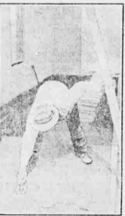
Photo by C. M. Barnitz. LAYING CONCRETE.
