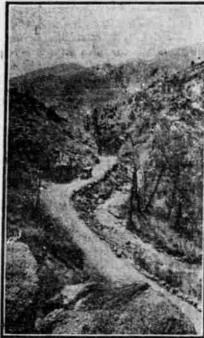
AN EXAMPLE OF A GOOD ROAD.
