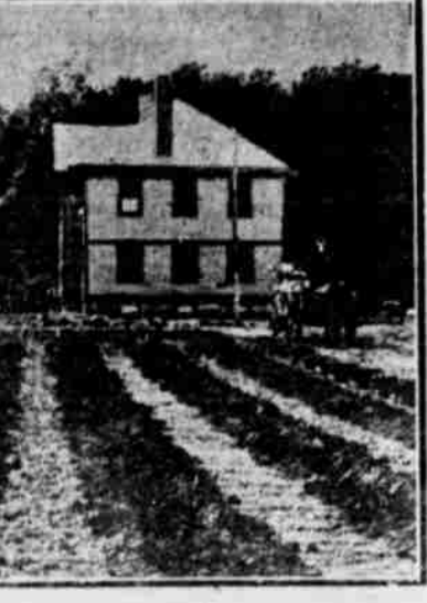
TRENCHED SOIL FOR WINTER WEATHER.
