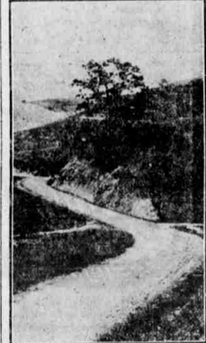
ONE OF COLORADO'S CONVICT MADE ROADS.
