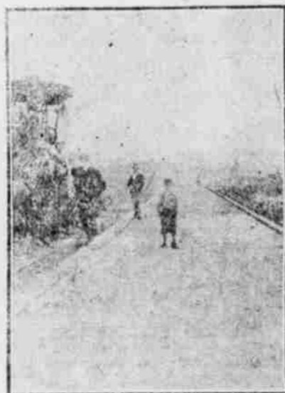
ALL READY TO LAY THE CONCRETE.
