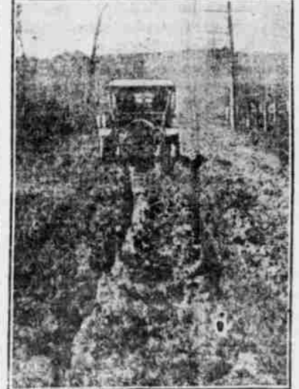
THE SORT OF ROAD WHICH CONVICTS ARE PUTTING INTO SHAPE.
