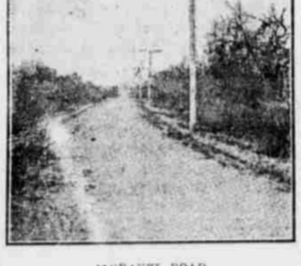
A GRAVEL ROAD.
