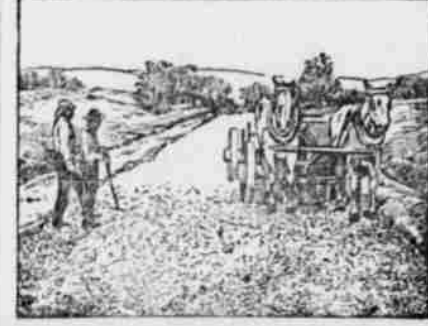
CONSTRUCTING A MACADAM ROAD.
