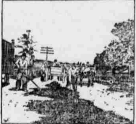
REPAIRING A ROAD.
