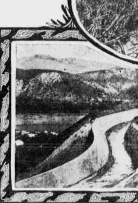
SLUICE GATE OF THE GOVERNMENT CANAL.
