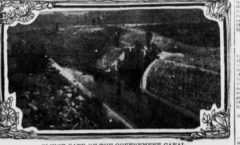
SLUICE GATE OF THE GOVERNMENT CANAL.
