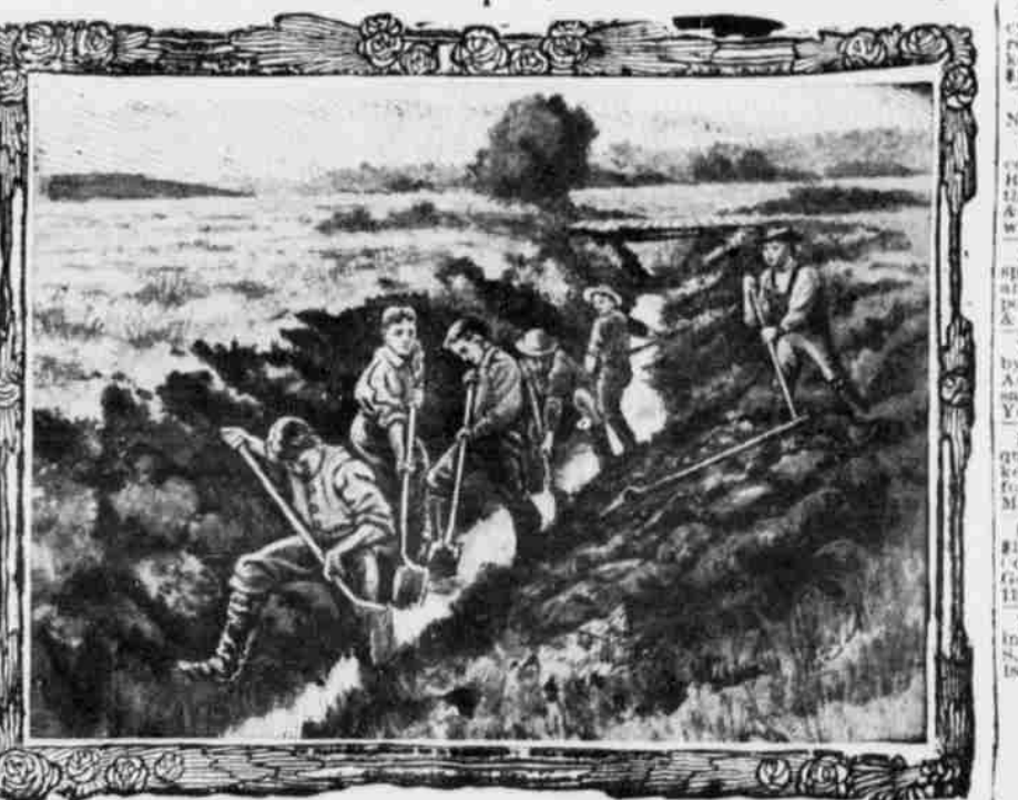
STUDENTS CLEANING OUT A DRAIN AT WINONA.
