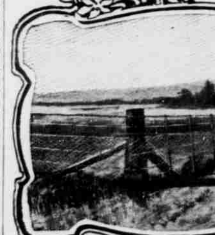
Fence Distorted by Improperly Placed Corner Supports
