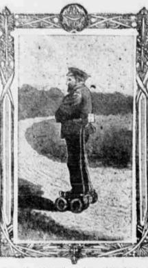
about the skater's waist. Attached to a tank are the lamition battery, the brottle lever and the spark control. A speed of 31 miles an hour can be attained and diminished by means of the throttle lever which the skater holds in his left hand. It is claimed that almost any hill can be climbed.
