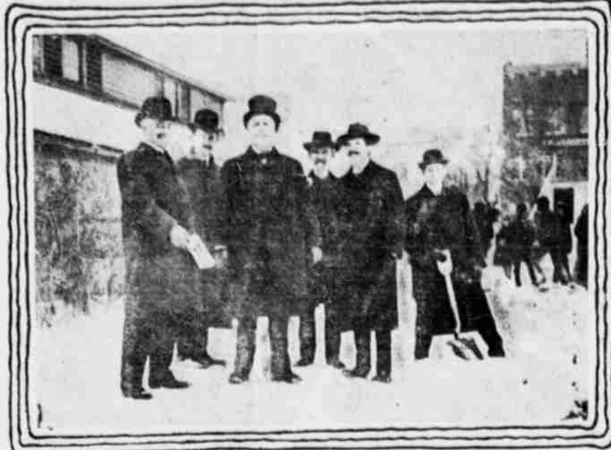
SECRETARY WILSON AND GROUP OF CHIEFS, DEPARTMENT OF AGRICULTURE GROUNDS AT TIME OF COMMENCEMENT OF WORK ON NEW BUILDING.
