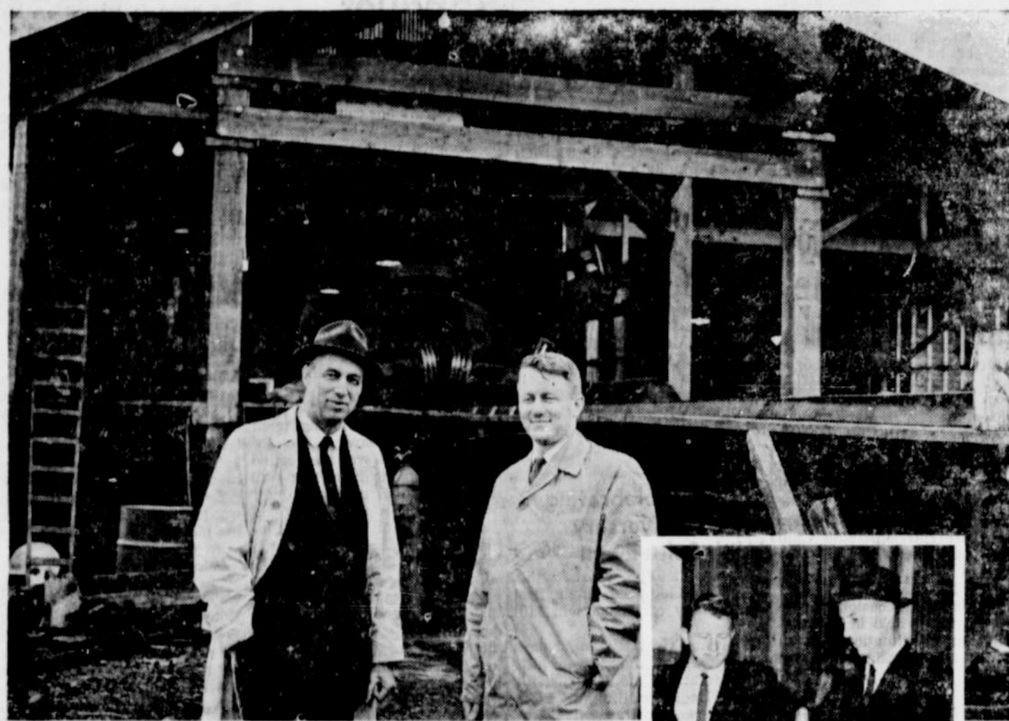
Mill Owner Ed Cone (left) and Bob Peterson, PP&L industrial development specialist, inspect electrically-operated barker installed as a result of PP&L study. Custom-engineered barker and chipper recommended by PP&L resulted in more efficient and profitable operation for mill. Besides running his mill, Cone performs an important civic duty by serving as mayor of Eugene. At right, Cone tests controls for new barking equipment.
