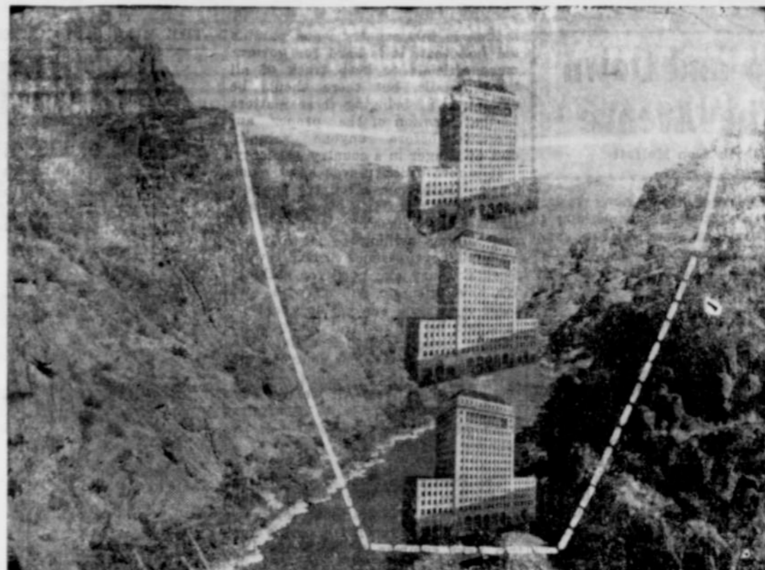
Pleasant Valley dam, one of the two huge projects included in $210,000,000 power development planned for middle Snake river, will be the third highest dam of its type in the entire world. Its giant concrete arch will tower 2½ times
