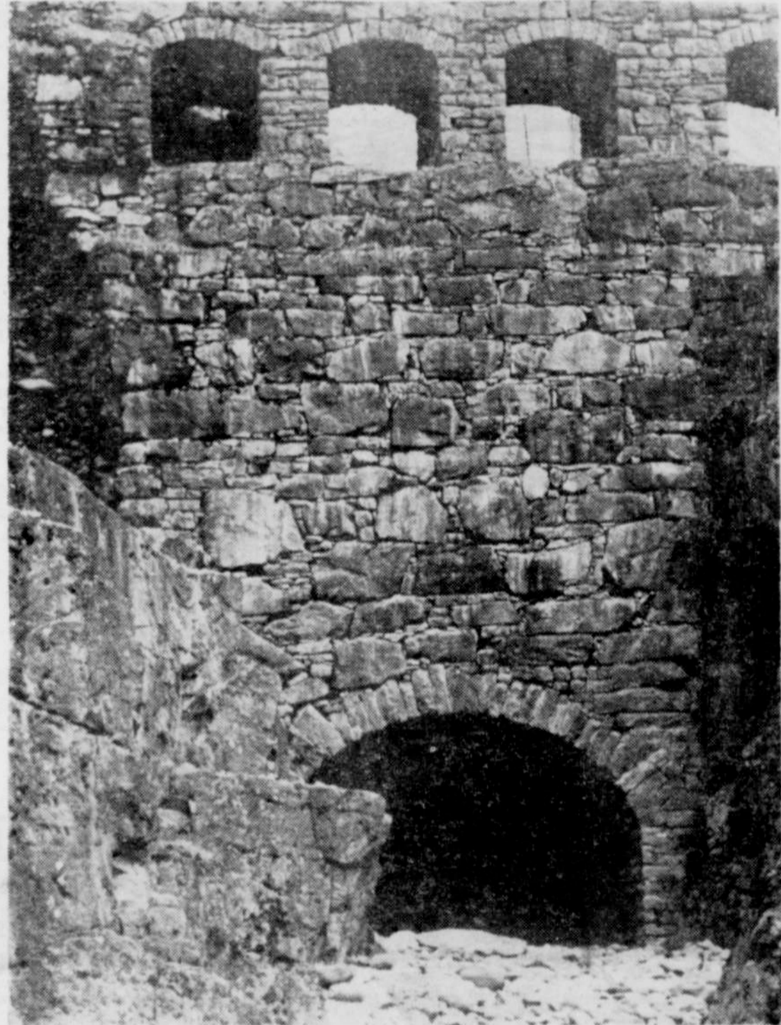
The North Santiam power project at Niagara, initiated by O'Neil brothers and Callaghan in the 1890s, was never dedicated because it was never completed. More than $100,000 was spent in a futile attempt to dam and utilize North Santiam water power where the stream is four feet and three inches in width during low water. (Photo courtesy Capital Journal)
