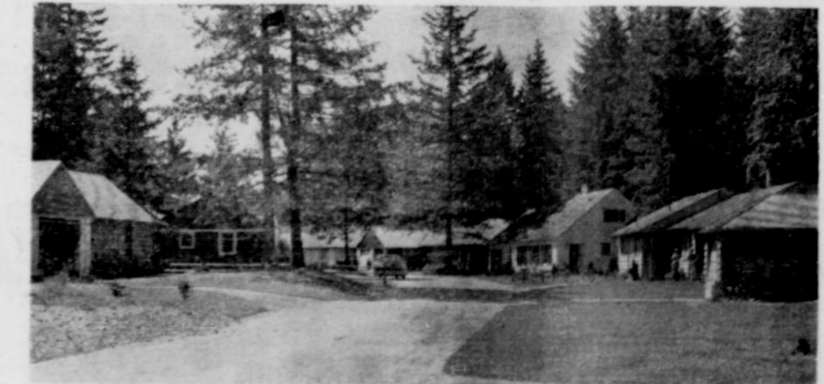
C.B.I., Detroit Dam contractors, housed their engineer personnel in these attractive Mill City homes in what is yet known as C.B.I. area or Kaiser Court. Army Engineers have purchased part of these homes for the personnel who will operate Detroit Dam. (Photo courtesy Capital Journal)
