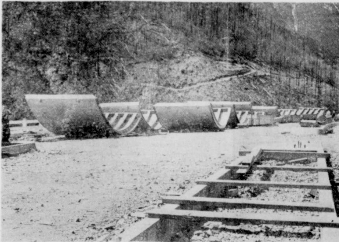
Massive spillway gates for Detroit dam have lately been delivered and are now being installed to bring the project to near completion. (Photo courtesy Capital Journal)
