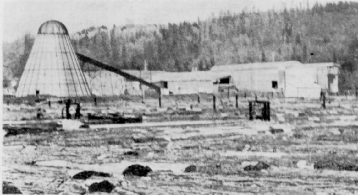
New $800,000 plywood plant of the M and M Woodworking company at Lyons which will open March 9. The 15-acre pond already is full of logs and a surplus of logs is being stockpiled for first production.
