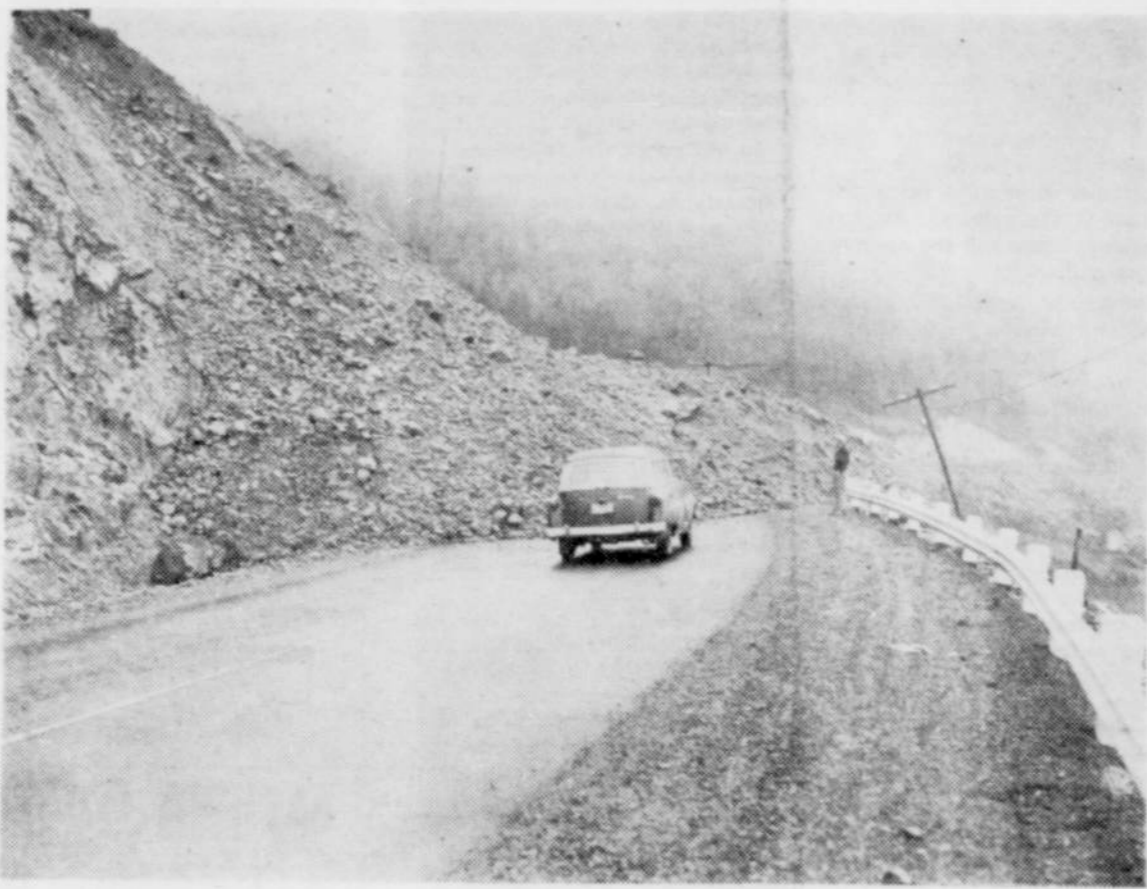
Huge rock slide on North Santiam highway that is expected to halt traffic for 10 days from both directions is shown with Sam Street, employee of the Bureau of Public Roads, inspecting the damage. The slide contains approximately 15,000 cubic yards of material and covers a 400-foot section of the highway about half a mile downstream from Detroit dam. (Photo courtesy Capital Journal and Robert Veness)
