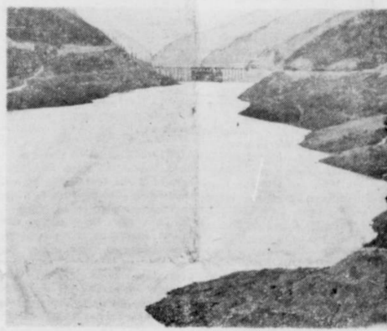
This huge volume of water impounded 250 feet deep back of Detroit dam, was prevented by engineers from roaring down the North Santiam river into the already flooded Jefferson area and causing major damage.
