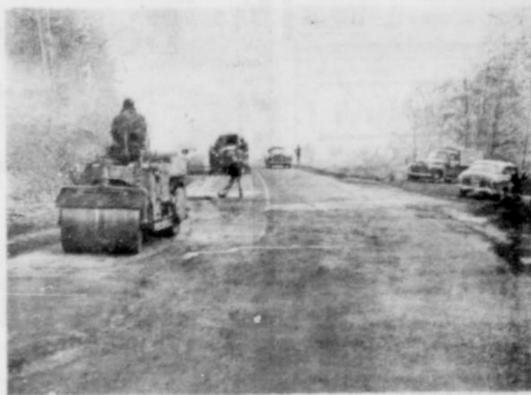
Tuesday state highway crews laid a final link of paving on the new scenic route between Fish Hatchery junction west of Mehama and Mill City. When an arch type, concrete bridge on the new route is completed within the next few days the road will be opened for traffic.
