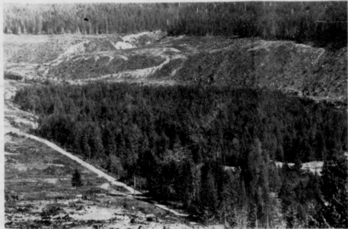
Inundated forest will become a Detroit dam catch basin—living trees shown in the middle section of this cleared area in Detroit dam reservoir will remain standing to become an inundated catch basin and filter for drift and sediment as water in the reservoir rises to a depth of 100 or more feet above their tops. Army engineers believe that such a natural catch basin will keep much water-logged drift, sediment and "floaters," too, from reaching Detroit dam.
