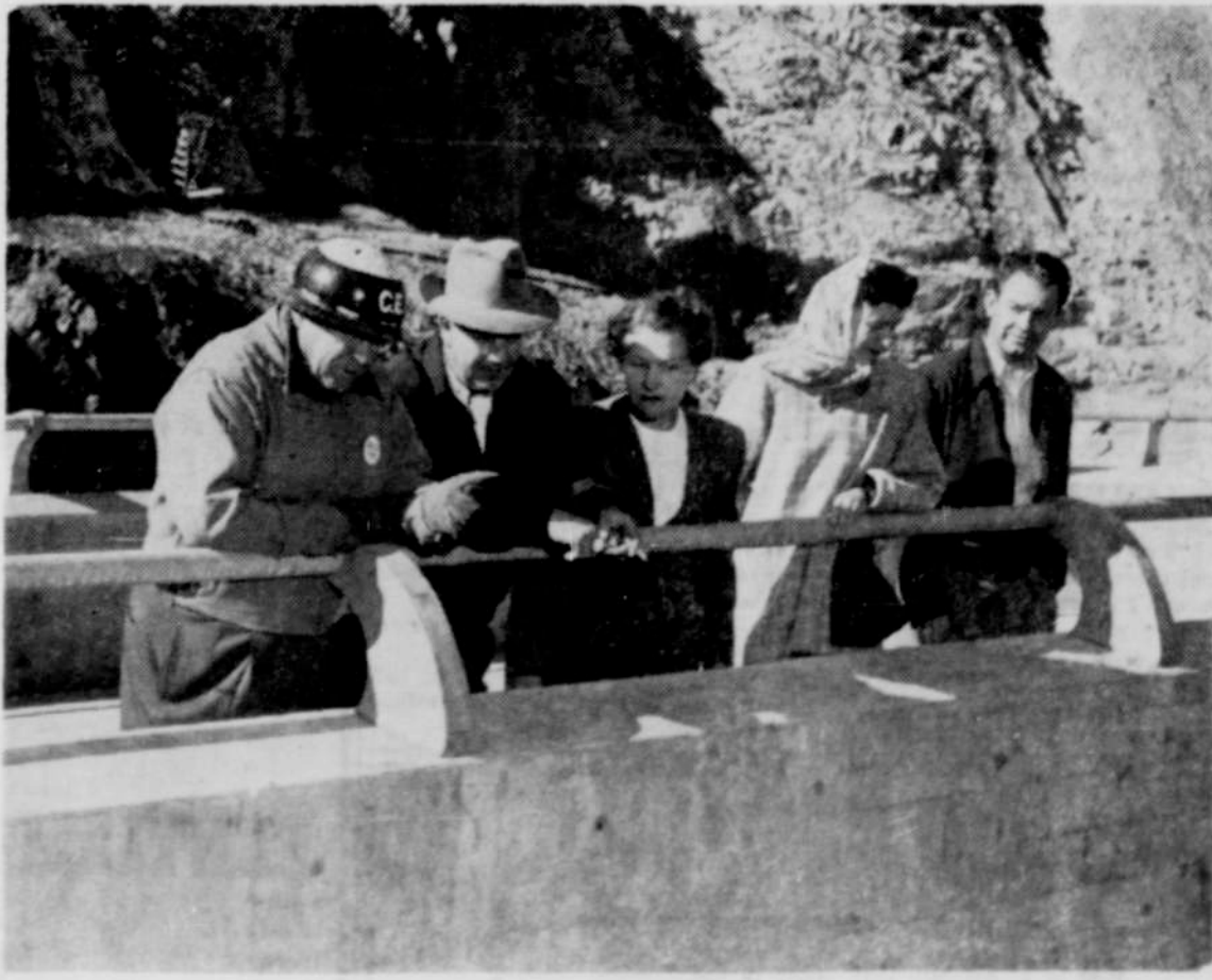
"Open House" at Detroit Dam—Pointing out features of the almost completed Detroit dam during "open house" ceremonies Saturday morning is (at left) C. W. Beck, chief of operations for the Corps of Engineers at the project. Among Mill City visitors for the special preview of the dam who heard Beck were Mr. and Mrs. Charles Lovell, Edith Veness, and Robert Hill, president of the Mill City Chamber of Commerce. (Photo courtesy of Capital Journal and Robert Veness)
