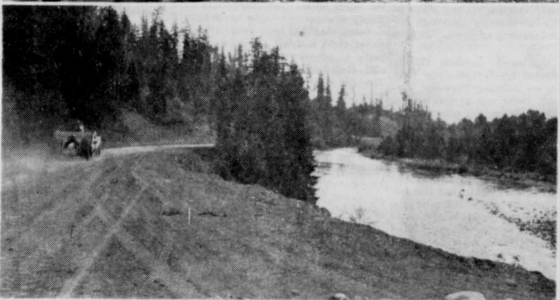
New North Santiam Route Approaches Completion—Top picture: Arch type concrete bridge 387.5 feet in length spans Little North Fork of the North Santiam two miles east of Mehama on the new route that will save .84 miles of driving between Stout creek and Mill City. Lower: Scenic attractions abound along new route where ballasting is now in progress. If paving is completed in October this pleasant, fast route may be open to public travel early this winter.
