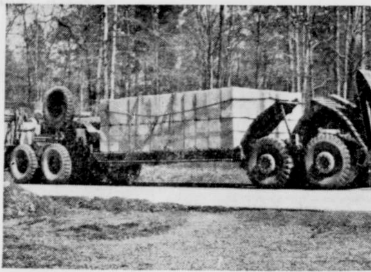
MONSTER TANK CARRIER TRIES TEST ROAD —This 200,000-pound Army tank retriever was one of the heavy vehicles used on the Maryland Test Road by highway engineers in an experiment which proved that pavement built on gravel will carry weights far greater than the heaviest commercial trucks permitted anywhere.
