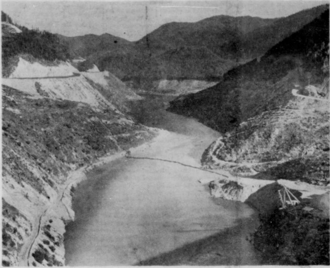
Waters of the North Santiam river slowly fill Detroit dam lake. Lake now stretches several miles upstream. North Santiam highway may be seen at upper left skirting highwater level of lake. Log boom to catch floating debris may be seen across lake in center of photo.
