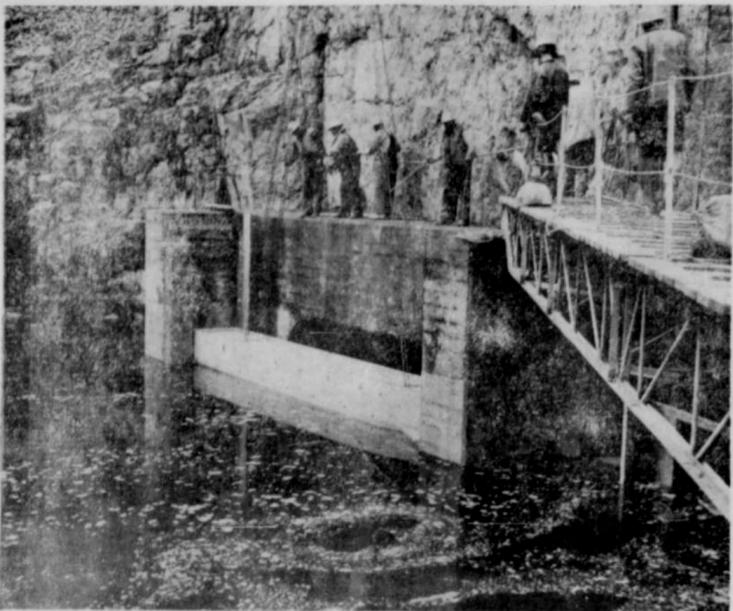
**STOPPER** Crews at Detroit dam on North Santiam river gently ease 18-ton slab of reinforced concrete into place at mouth of diversion tunnel. Fourteen of slabs were used to plug tunnel through which river flowed two years. Second man from right holds telephone to direct crane operator atop cliff. At right is intake of temporary bypass tunnel.
