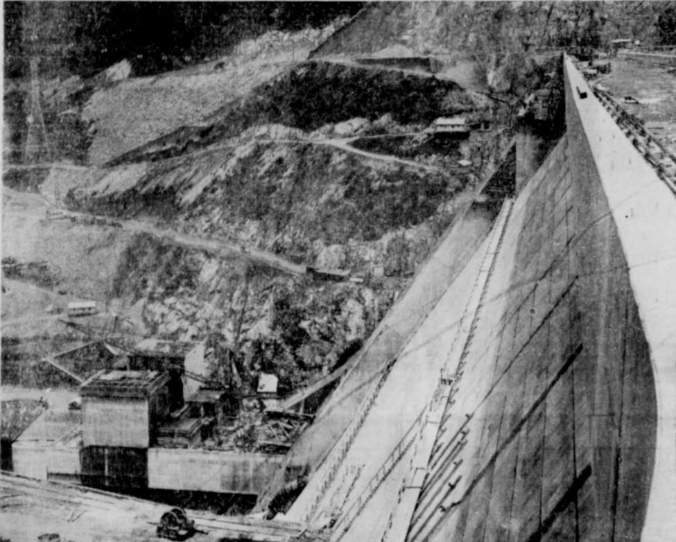
**PANORAMA** View of Detroit dam on North Santiam shows highway across top, partially complete powerhouse (left at river level) and main highway grade
