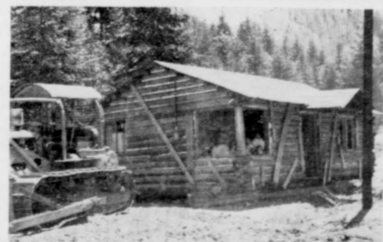
One of the last homes to be moved from the Detroit reservoir area was that of Mr. and Mrs. John Bryant. Photo shows the house on skids being moved up a back road to a new site near Breitenbush river. Mrs. Verry Johnson and Mrs. Bryant may be seen in the windows occupying it on the journey up the hill. Children with them are Evelyn Harper, Allen Johnson and Jane Johnson. Deadline for moving was midnight Monday. (Photo courtesy Capital Journal)
