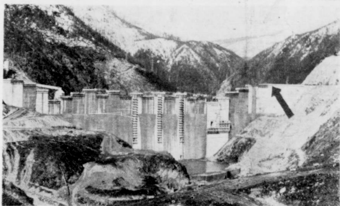
The picture above shows the present state of construction of Detroit dam. When the dam is completed the top will be on a level with the point indicated by the arrow. The dam will be 463 feet high from foundation to deck, 1579 feet above sea level, and will be 1580 feet long. Maximum width at the base will be 335 feet. (Photo courtesy Capital Journal)
