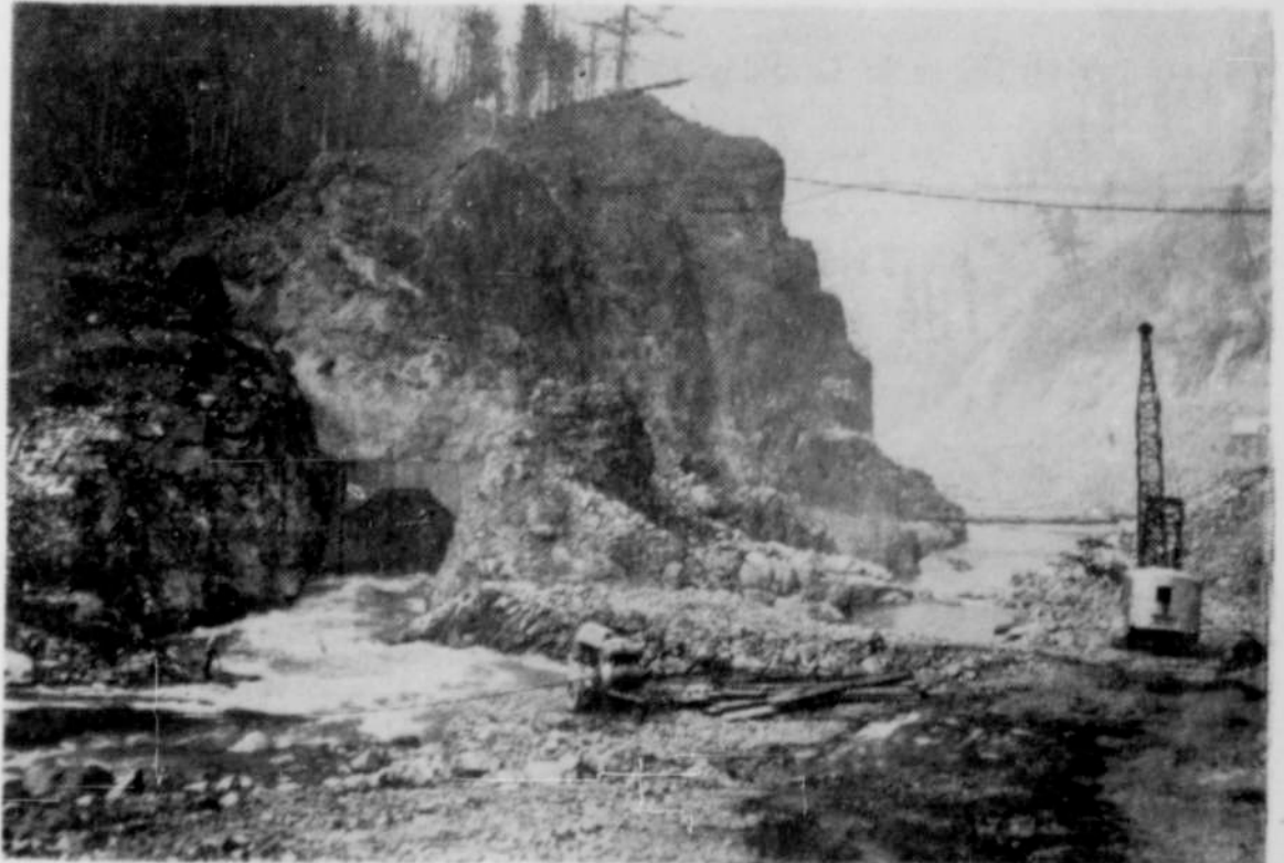
This is Big Cliff dam's diversion tunnel as seen from an upstream vantage point on a level with the bed of the North Santiam river. The temporary coffer dam of rock can be seen in the center of the picture as it connects up with the mouth of the diversion tunnel. A foot bridge across the river bed can be spotted near the power crane in the picture. Water is now flowing through the completed Big Cliff diversion tunnel. Work on the main dam is now underway. The concrete structure will rise within that area defined by the power cable strung across the chasm shown to the right. (Photo courtesy of the Capital Journal)
