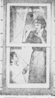
PITTSBURGH --- The new Flexseal Bomb Glass units open automatically in four triangular sec-tions when an explosive force strikes. This release of pressure prevents the window frame from being blown in and greatly reduces the possibilities of flying fragments. The window consists of three lay-
