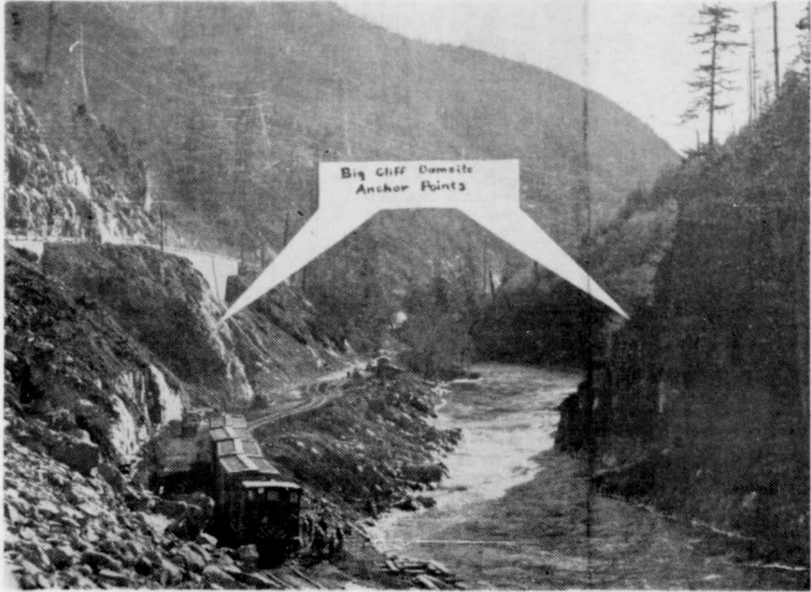
Looking downstream from highway 222 alongside the North Santiam river towards Mill City near Big Cliff dam. One can see the bare rocks that rise steeply above the bed of the river and that will shoulder the load of Big Cliff dam. Recently Army Engineers let a contract for turbine governing equipment and spare parts for this dam. Wednesday Army Engineers accepted the bid of R. H. Jones of Hillsboro for clearing of Big Cliff dam reservoir area. Big Cliff dam is scheduled as a constant flow regulatory unit and as a power producer. (Photo Courtesy of Capital Journal and Bob Veness)
