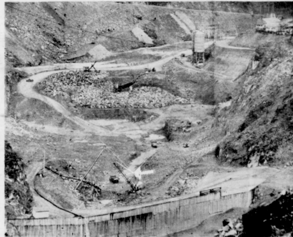
Seven months of concrete pouring on Detroit Dam places the spell of a magic wand over a once yawning chasm. Above, 350,000 yards of concrete, one-fifth of Detroit Dam, now squats solidly where once there was no shaped concrete—just nature. The white arrow in the picture below marks the resting place of the first bucket of concrete poured on August 5, 1950. (Photos Courtesy of Capital Journal)
