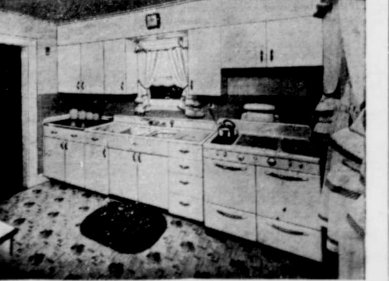
Symbolic of the transformation is the electric clock that replaces the old mantel timepiece. Alterations? Sure, but not expensive ones, because standard steel kitchen units were used and no structural changes were made. The window remains and the new cabinet sink was attached to the old plumbing. A soffit above the wall cabinets and the addition of wall tile are extra features. Note the large number of drawers and compartments in the double-bowl sink and base cabinets.
