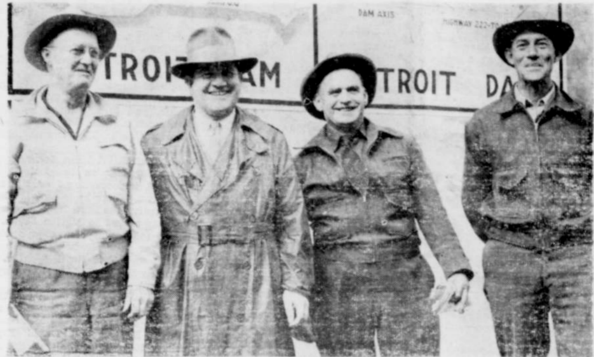
Somewhat prepared for rainy weather, Mill City's jacketed industrial committee members of the chamber of commerce delegation met the Willamette River Basin Commission caravan at the Detroit damsite on June 24. Also greeting the touring group was C. C. Davis, resident engineer for the dam. Pictured from left to right are George Veteo, Davis, C. E. Coville and C. F. Hunter. (Picture Courtesy of the Capital Journal)
