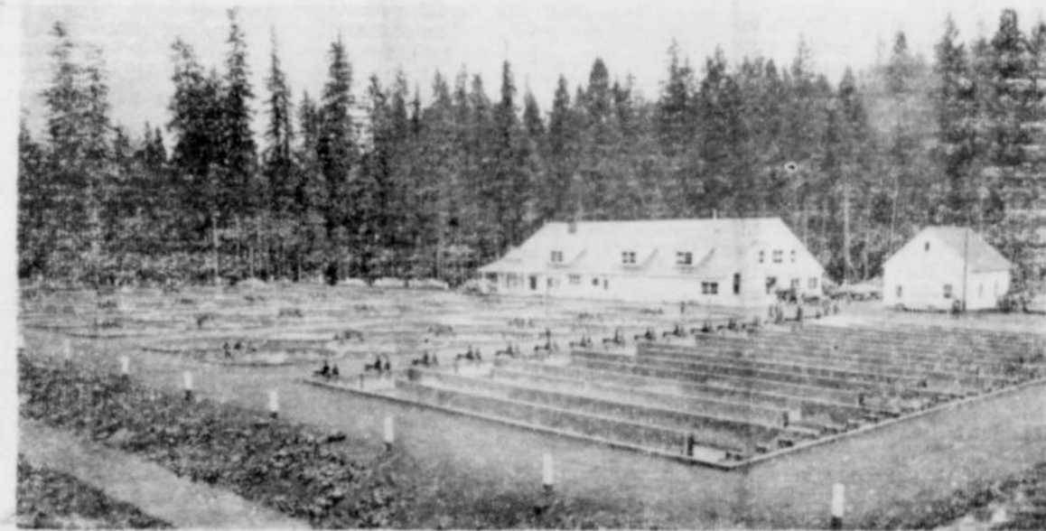
One of the upper canyon's newer landmarks is the Marion Fork Fish Hatchery above. Regarded as the second largest fish hatchery in the northwest, the Marion Forks plant will cost more than $800,000. Here fish eggs transported from below Detroit Dam will be handled in a unique attempt by the state fisheries department to overcome the lack of fish ladders at Detroit Dam caused by the tremendous height of the structure. Fishing authorities are closely watching the Marion Forks hatchery program to see if fish can be successfully handled in this manner. A shipment of fish from the Mehama hatchery in a few weeks will begin operations. (Picture Courtesy of the Capital Journal)
