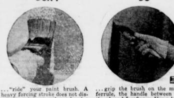
ferrule, the handle between the thumb and forefinger. Use a long, steady, even stroke, lifting the brush gradually at the end of the stroke to feather out the edge.
